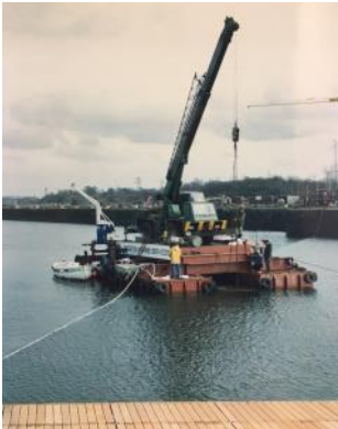
January 1990 - installation of the pontoons using a specially constructed crane barge.
